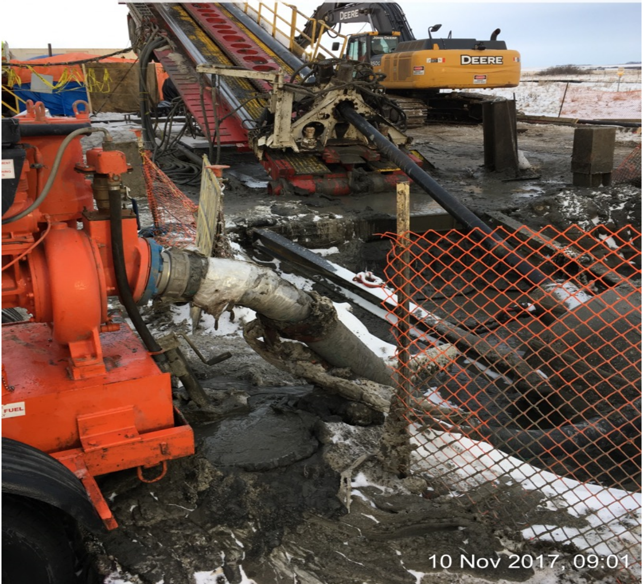
HORIZONTAL DIRECTIONAL DRILLING AT SOUTH SASKATCHEWAN RIVER
