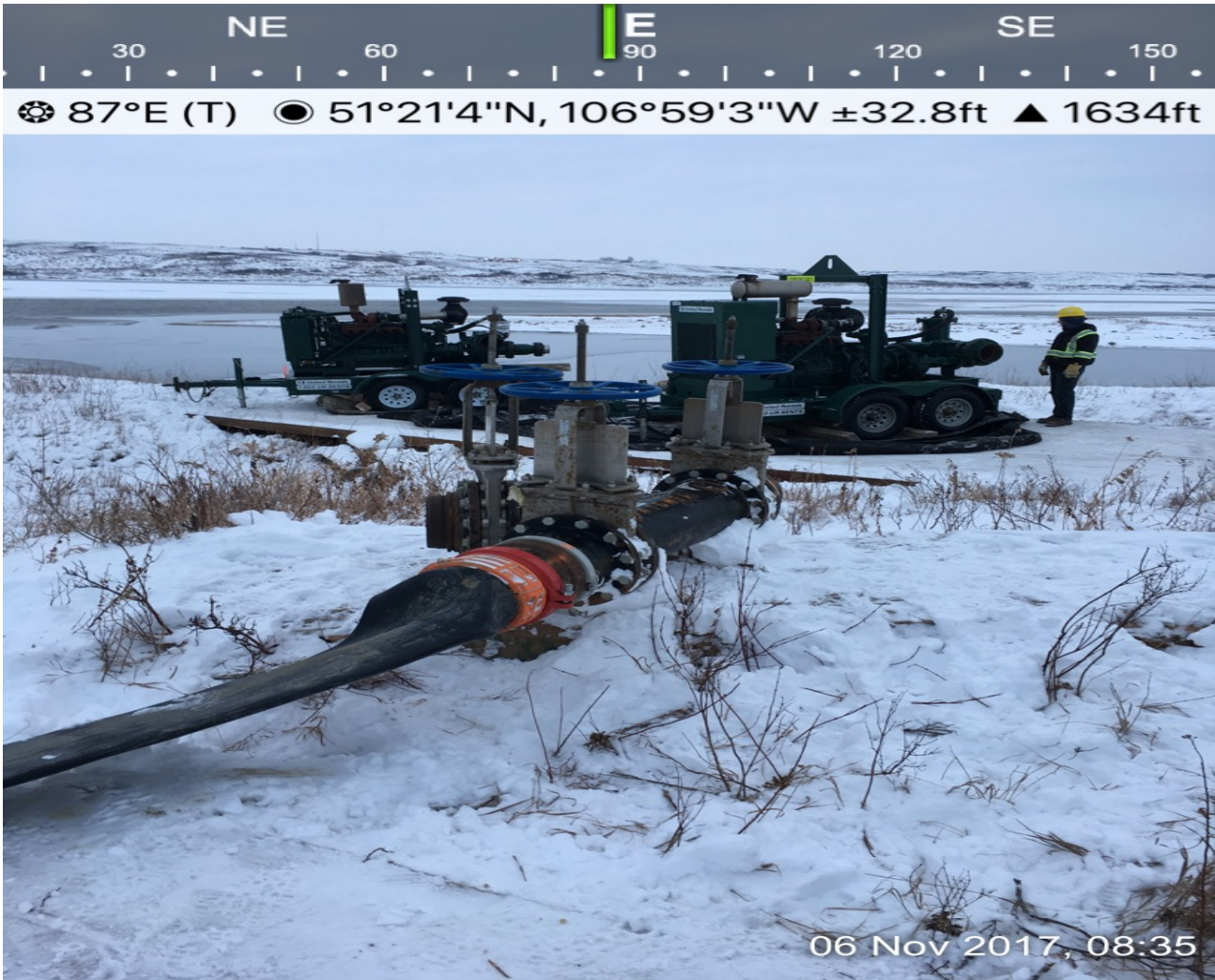
PUMPING WATER FROM THE RIVER INTO THE MAINLINE
