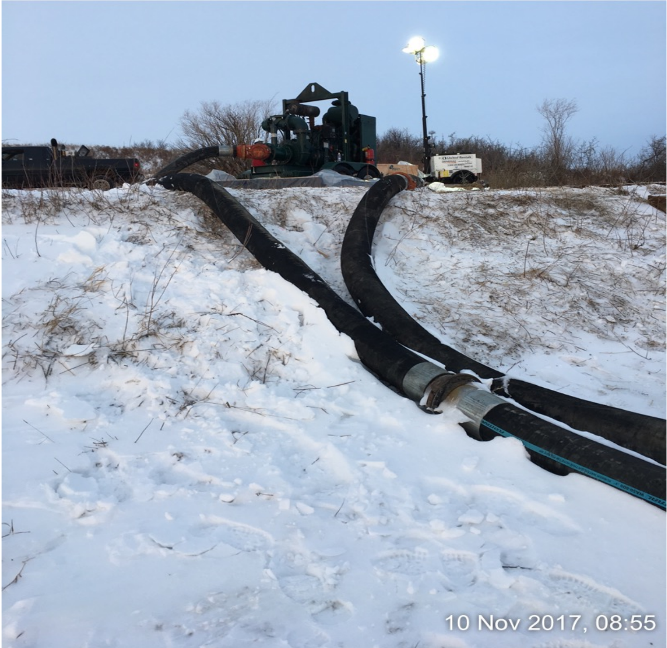
PUMPING WATER FROM THE RIVER INTO THE MAINLINE
