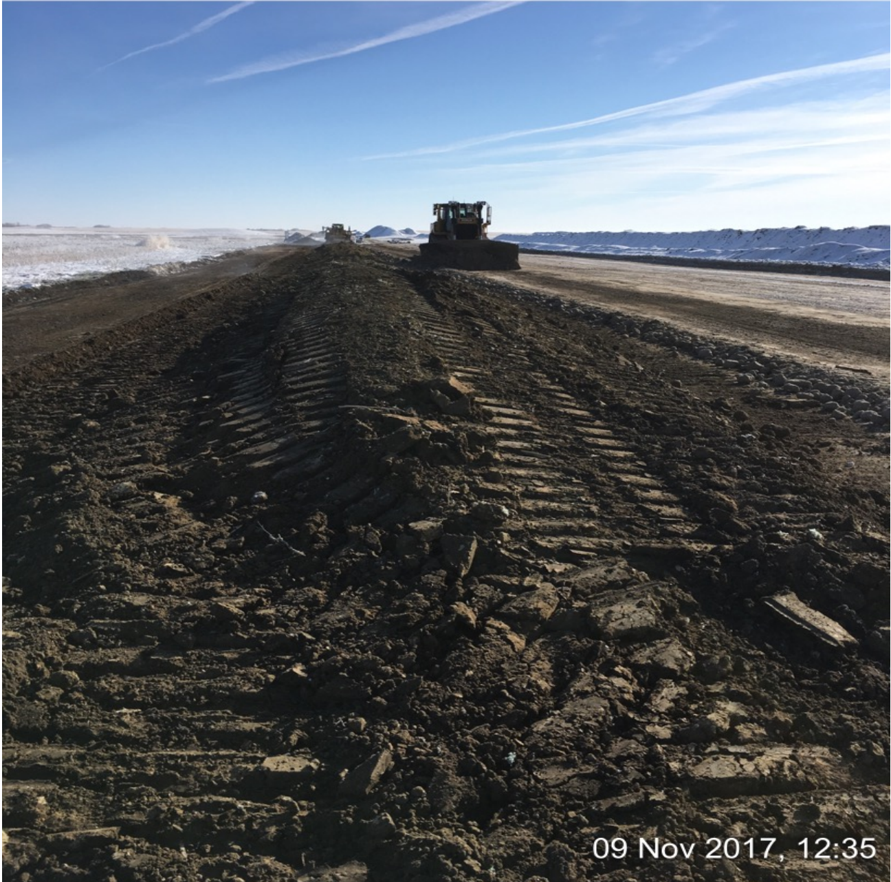
LAST STEP OF THE BACKFILL PROCESS
