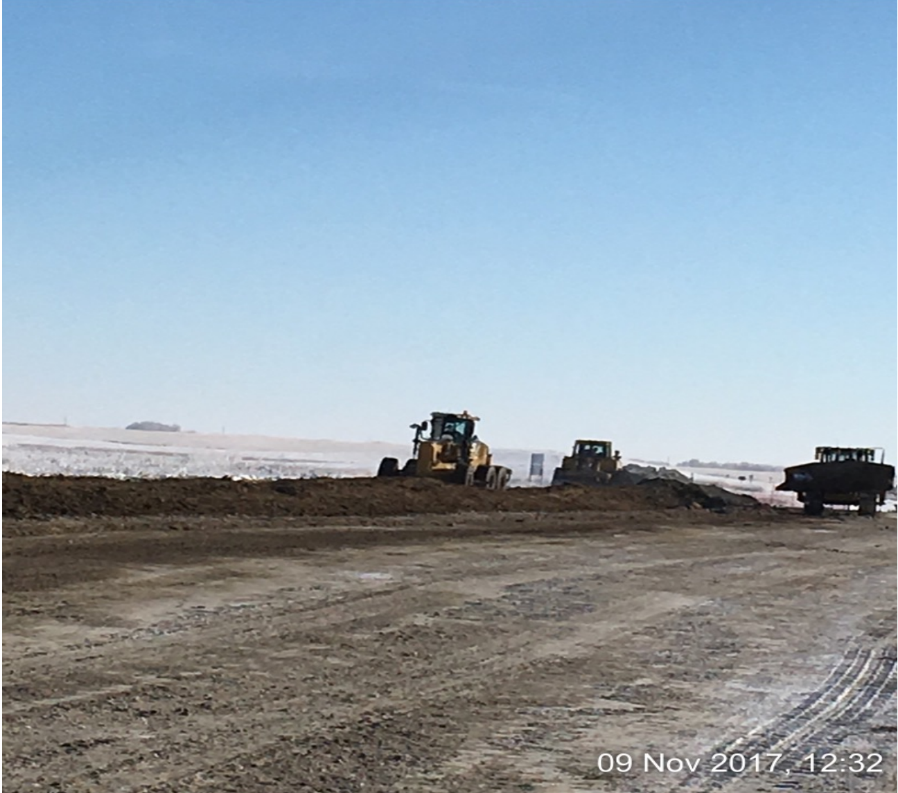
BACK END OF BACKFILL CREW
